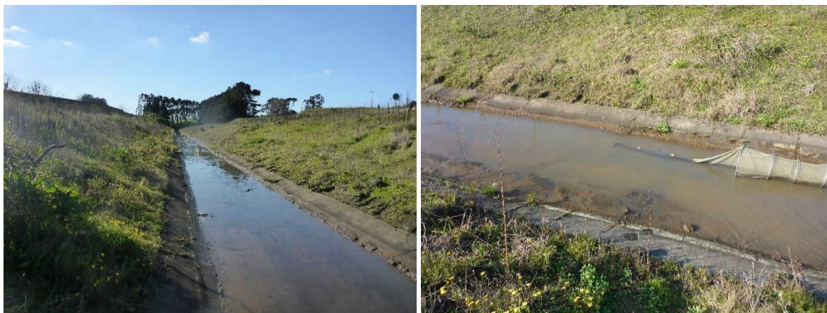
Photograph 5.2: Typical channel at Site B, North Drain (no flow from Dewatering Plant at time of photograph).
